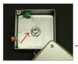
2. Insert ceiling mount through ceiling tile hole, and into JBM40 box then tighten the knurled nut.
